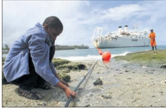
**SHORE LANDING:** A worker checks an undersea cable at its beach base. The cables form a vital part of the communication chain.
